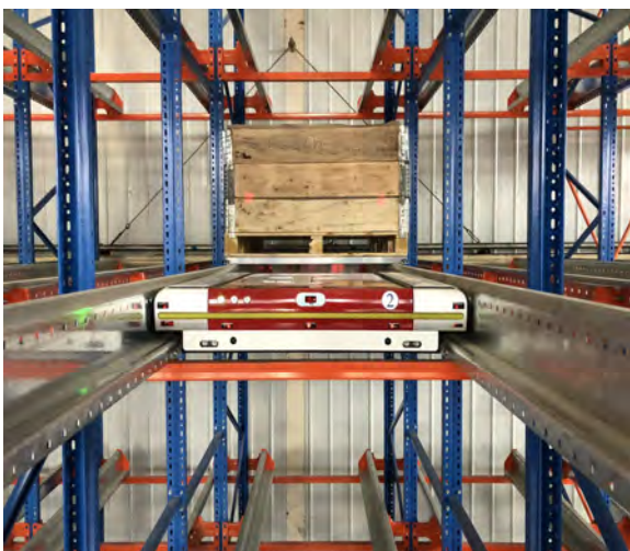
Tianjin Stacker Project (fork type)
